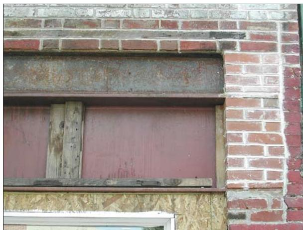
Fourth, the oriented strand board (OSB) sheathing at the bottom of the photograph shows that there is combustible construction in this building; that is additional fuel for a fire.
