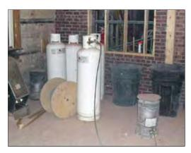
Cylinders and the valve-protecting devices should be arranged to minimize the likelihood that escaping gas from the pressure relief device will impinge on the cylinder or adjacent cylinders. Heating appliances must be at least 6 feet from any cylinder. Blower- or radiant-type heaters must not be directed toward any cylinder within 20 feet of the heat source.
